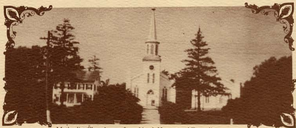
Methodist Church seen from North Hempstead Turnpike.
